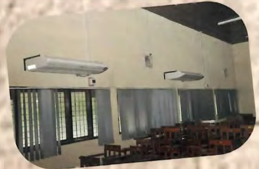
Air Condition Project
